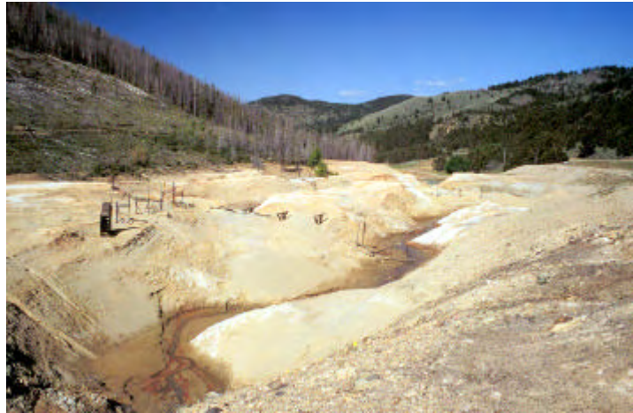
Figure 1 -Comet Mine prior to Phase I reclamation.
