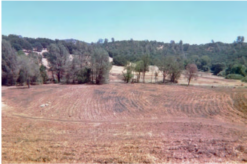
Photo 18 - Final site grading – note that filled mine pit is in center of photo
