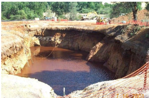
Photo 4 - Mine pit dewatering, July 16, 2001
