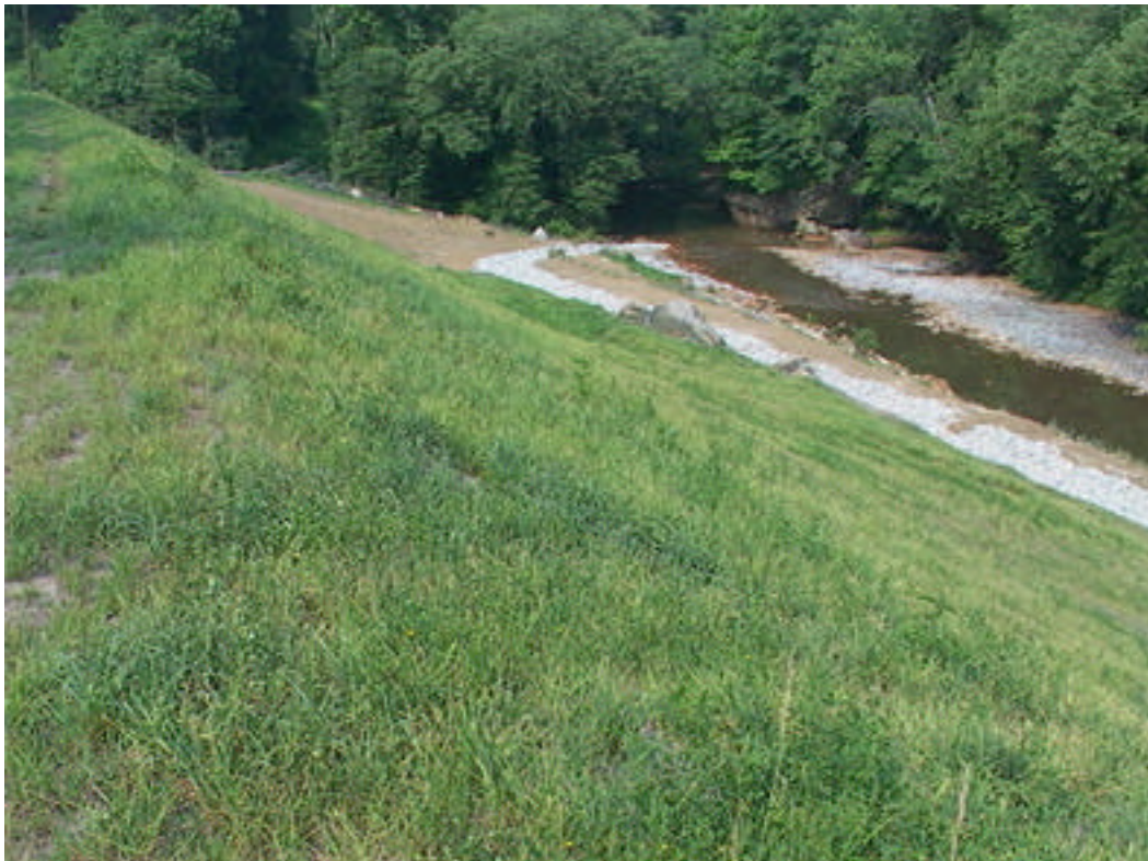
Figure 12. Water Tank Hollow Refuse Area after reclamation.
