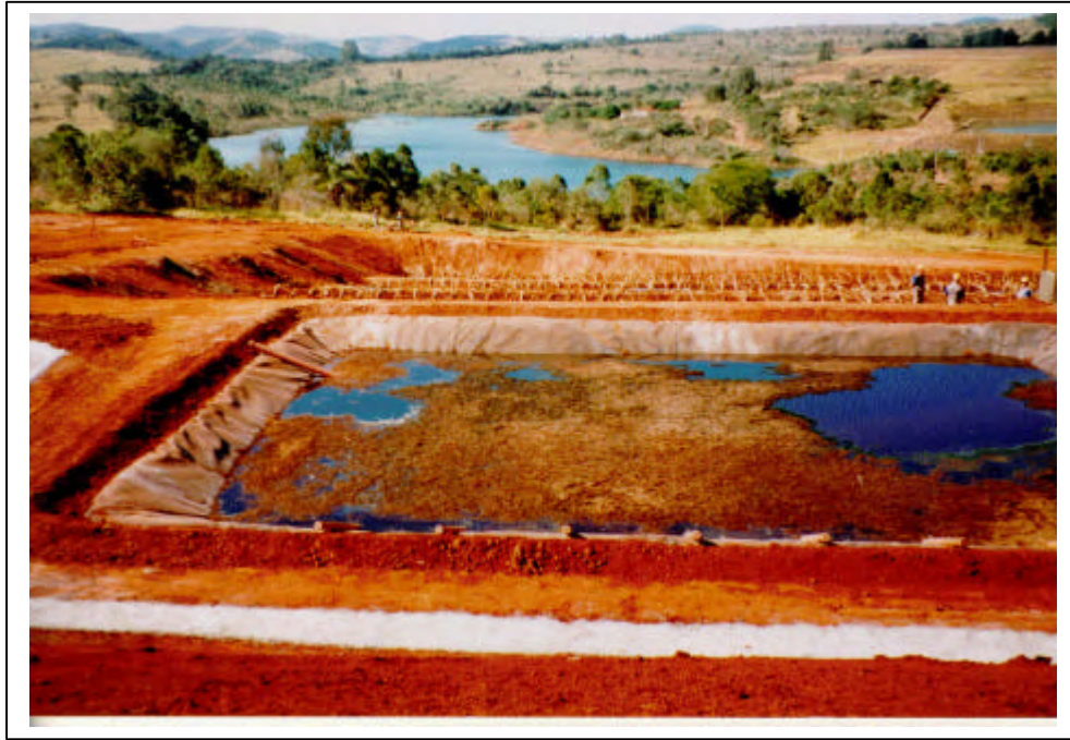
Figure 3. A Typical Sulfate-Reducing Bioreactor
