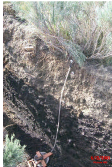
Picture #6, Pit #4 south side Compacted Refuse
