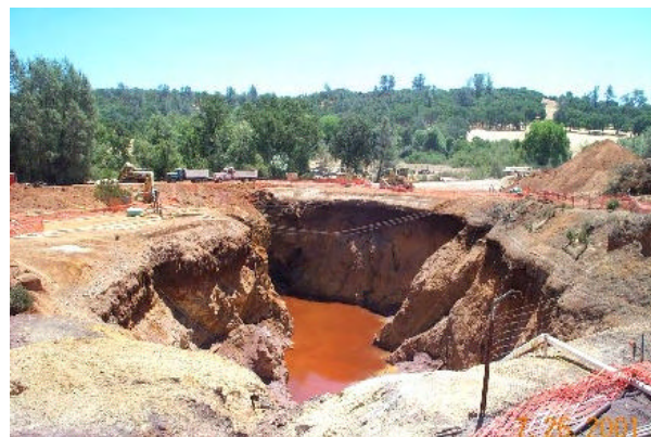
Photo 5 - Mine pit dewatering, July 26, 2001
