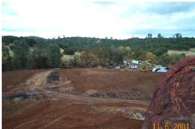
Photo 14 - Placement of soil cover
