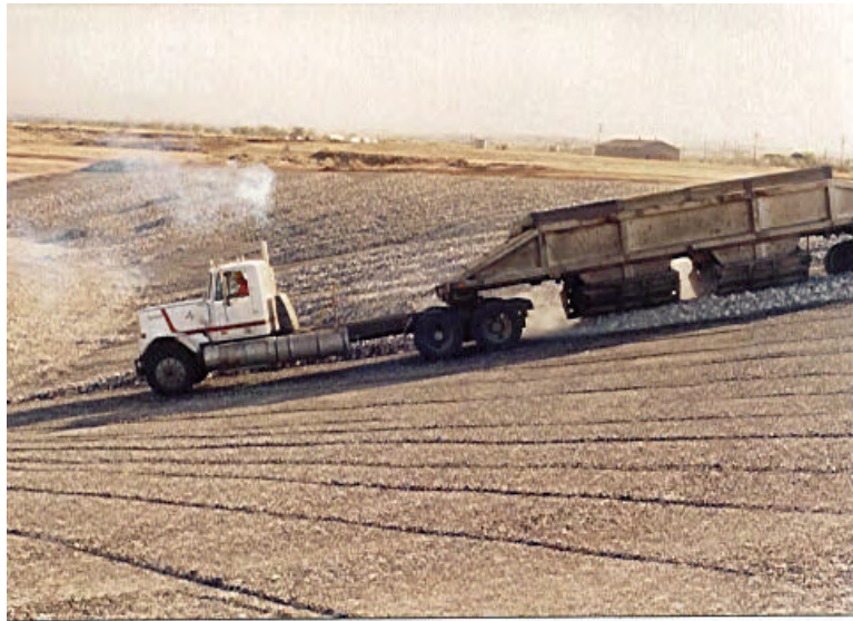
Rock placement on asbestos disposal area
