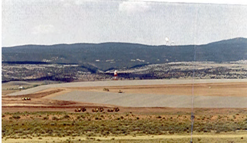
View of Stabilized Impoundment Slope
