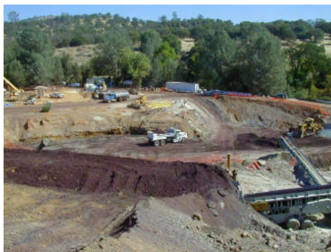
Photo 11 - Mine waste placement with trucks and dozers
