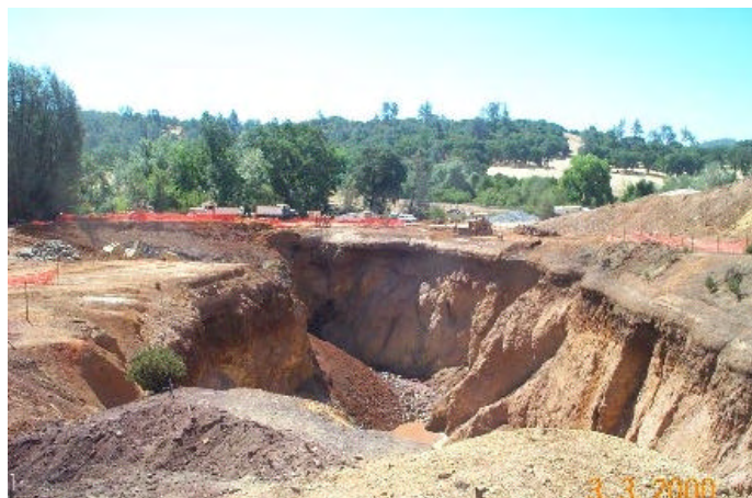
Photo 8 - Pit access ramp
