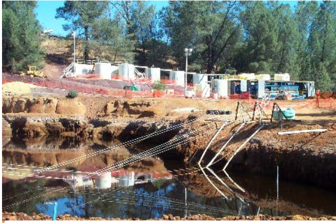
Photo 7 - Treatment plant and pit dewatering
