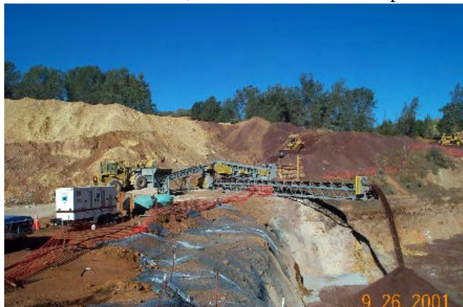
Photo 10 - Mine waste placement with conveyor
