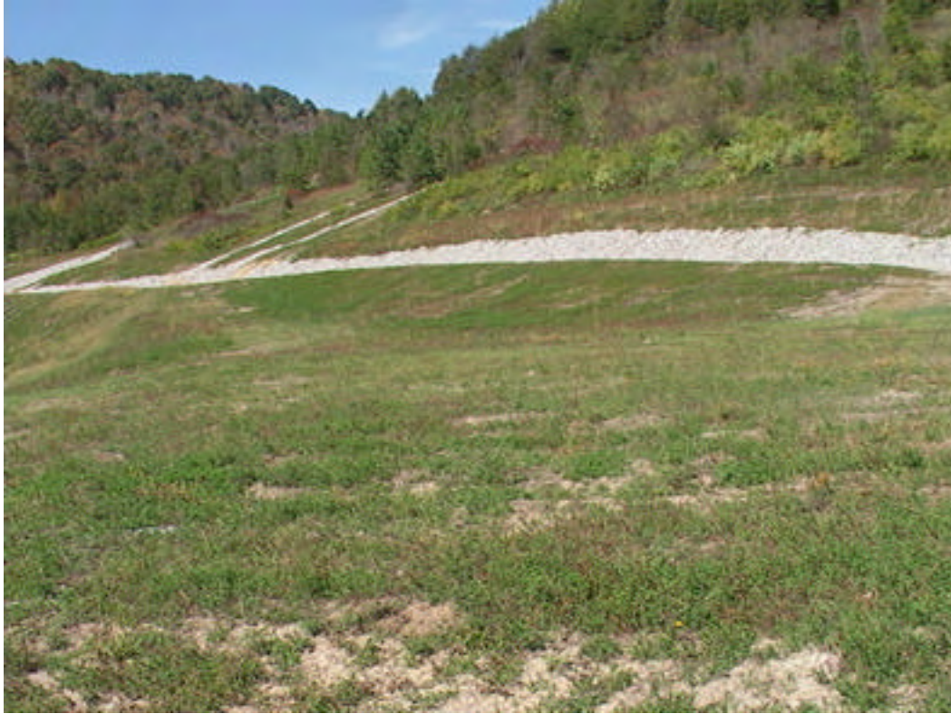
Figure 13. Roberts Hollow Refuse Fill Area after reclamation.
